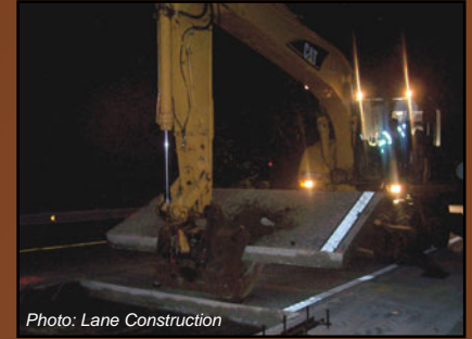
Photo: Lane Construction
