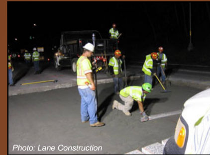
Photo: Lane Construction
